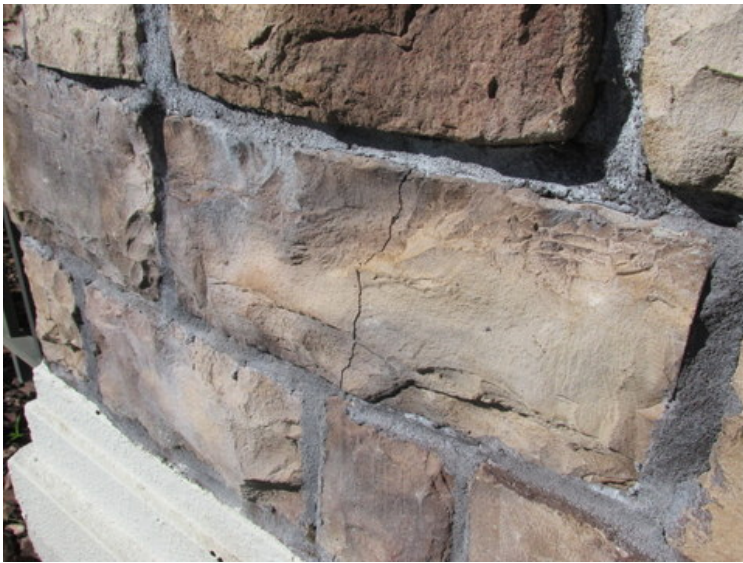
Masonry crack
