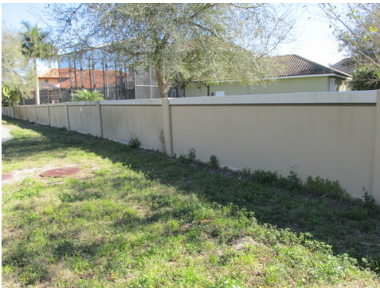
Stucco perimeter wall
