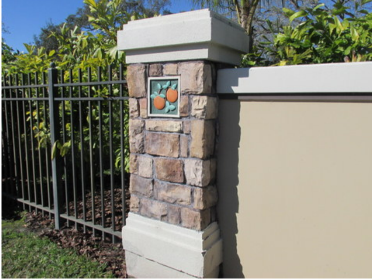
Masonry column at perimeter of community
