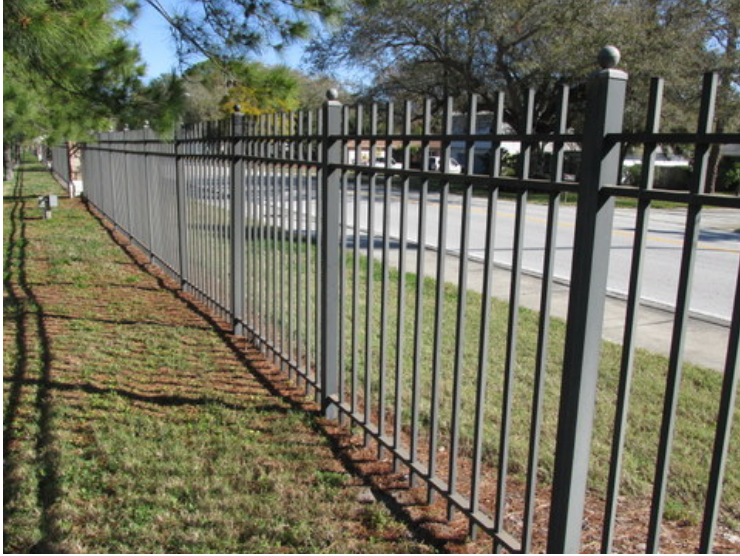
Aluminum perimeter fence
