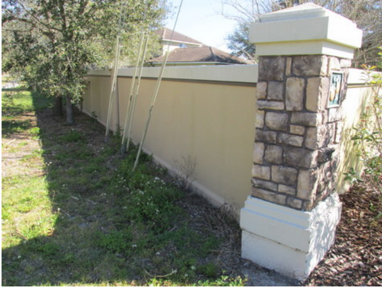
Stucco perimeter wall
